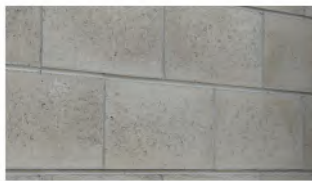
CONCRETE BLOCKWORK FAIR FACED BLOCKWORK
